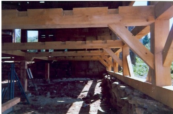
Fig. 2: After restoration with new hemlock frame
