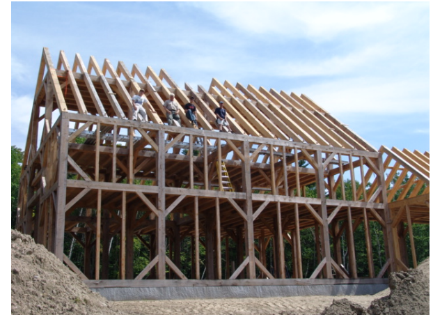
Fig. 3: New timber frame
