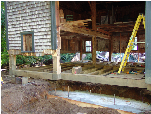
Fig. 6: This is the same barn showing the post-bottom repairs
